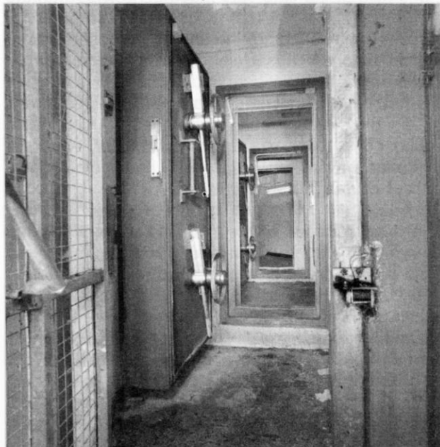
The 'Clean' entrance into the bunker with its steel and concrete blast doors. Photo by Nick Catford
